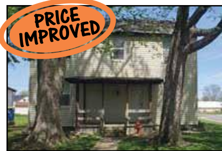
3 bedroom, 1 bath, home located on a spacious corner lot in the heart of Aviston! There's a 17 x 17 storage building as well as a oversized two car detached garage with alley access and concrete driveway! 99 East 3rd Street, Aviston $119,900
