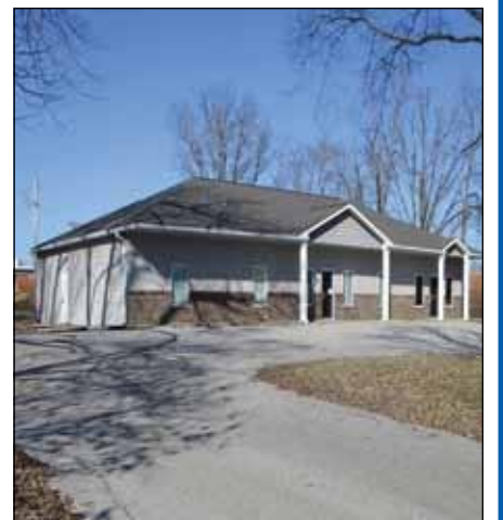
Well known Professional Retail building on Walnut High traffic area. 206 Walnut Street, Highland $460,000
