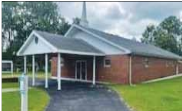
Covered entry way, 3000 sq ft church. Garden shed included. Selling "as is". 109 College Street, Alhambra $175,000
