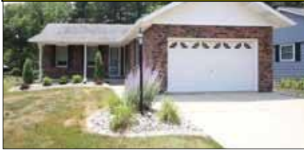
Well maintained all brick custom home with vaulted ceiling, wood floors, gasp fp, island in kitchen, finished LL, oversized 2 car garage. 5 Trout Drive, Highland $259,900
