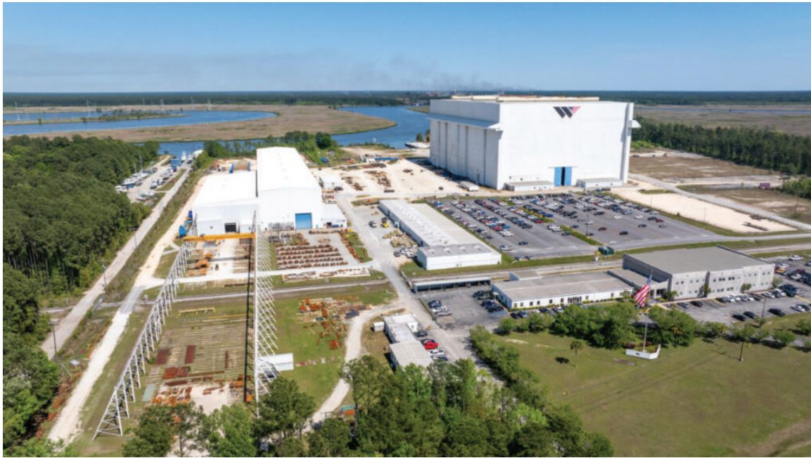
The former W International metal fabricating site in Goose Creek is the subject of an $80 million whistleblower lawsuit unsealed Monday in federal court in Charleston. The company's assets were acquired last year by Navy contractor Newport News Shipbuilding. This photo is from the company's January 2025 announcement. (Courtesy of Huntington Ingalls Industries)
