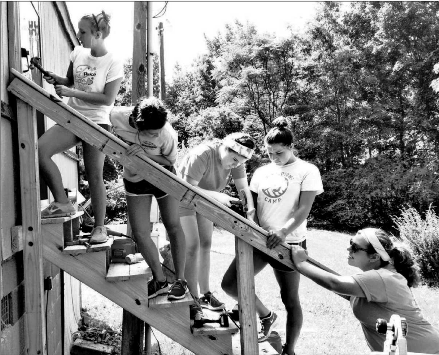
These Youth Serve volunteers took a multi-step approach to starting repairs on this home during last week’s youth ministry. From the top down are: Laykin Bowers, Bridget McKinney, Rachel DeBruhl, Taylor Barrett, and Sydney Phillips Photo provided.
