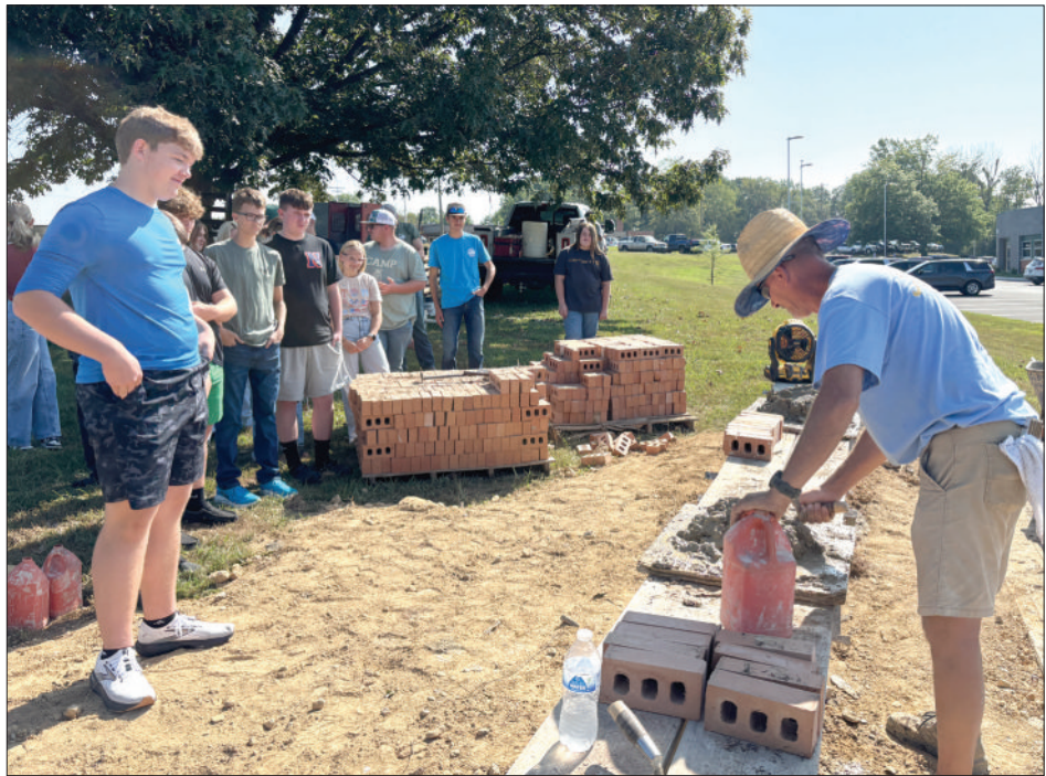
The fall Ag Construction class went to watch Matt Goodin and his employees construct the new GCHS sign.
