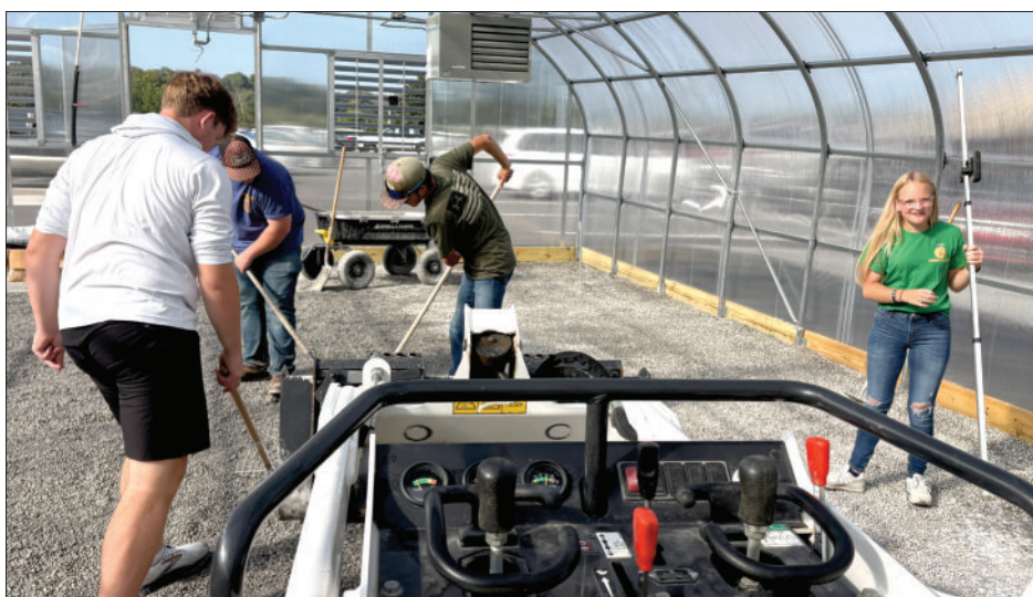
The Ag Construction class were leveling rocks for the construction of the new greenhouse.
