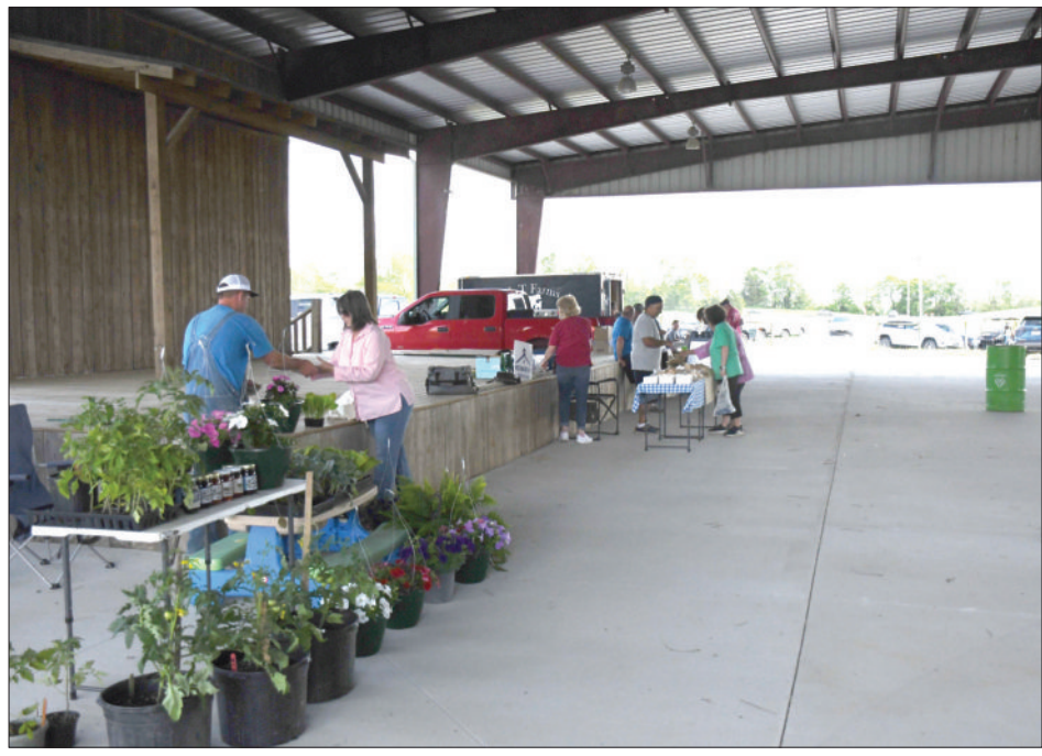
Lots of improvements have been made to the Cattleman's Pavilion where the Farmers Market takes place each Thursday afternoon. A concrete floor has been added. One corner of the building has been enclosed and more floor space has been added to the facility.
