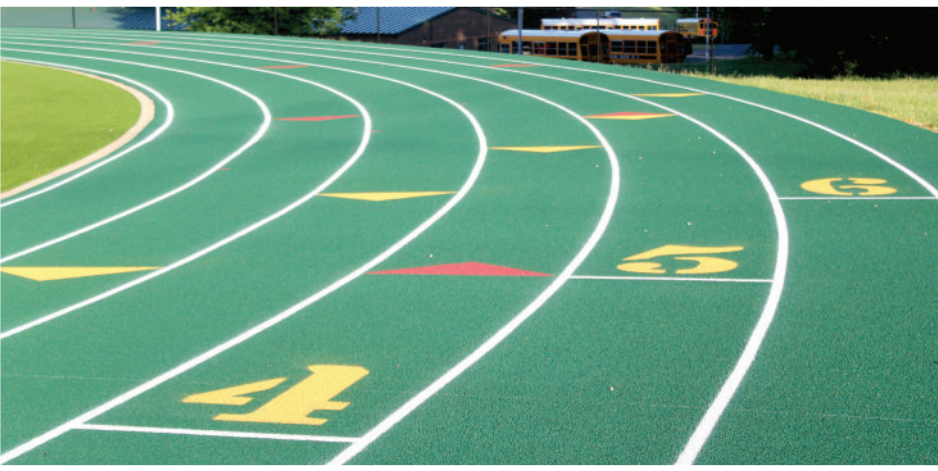
Green and gold! The marking and numbering of lanes added to the track's attractive appearance. Work on the track at Dragon Stadium began in early April and was recently completed. It involved repairing a damaged area, the spraying of a primer coat and two structural spray coats, along with installing lane lines and event markings in accordance with KHSAA/NFHS standards.
