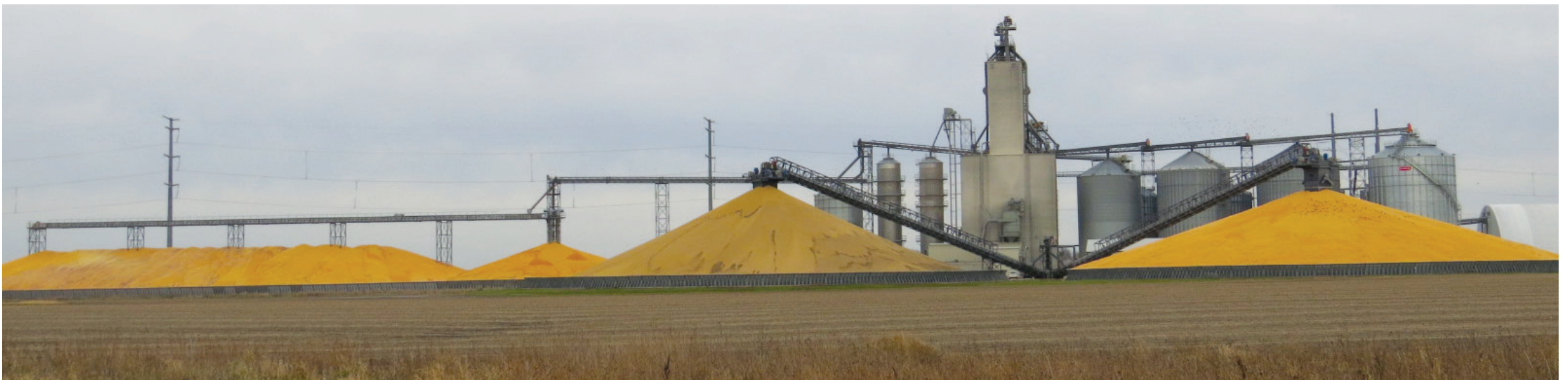
Evidence of a big crop in 2025 was shown in the outdoor storage at the Agassiz Valley Grain Terminal north of Barnesville. Several million bushels of corn and soybeans were stored in outdoor bunkers to be picked up and shipped over the winter on westbound unit trains.
