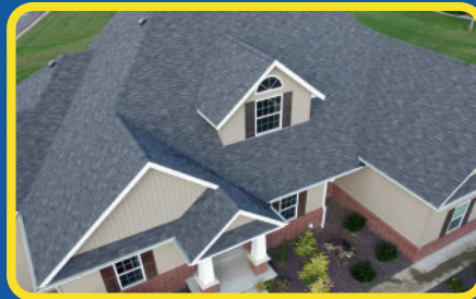
Roofing, Siding, & Gutters
