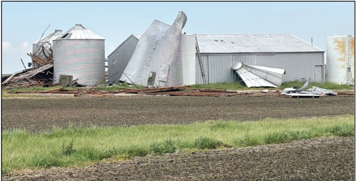
Damage at the Streitmatter Brothers farm in rural Sparland
