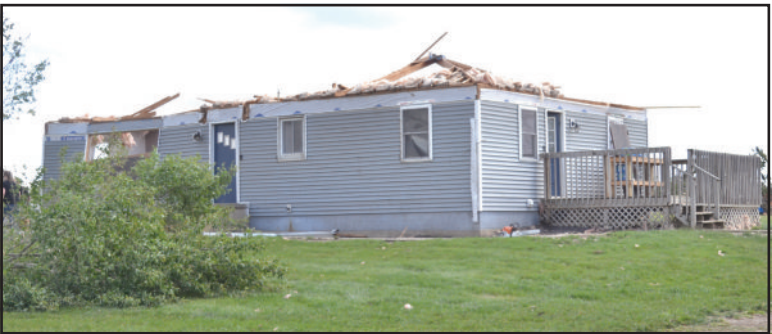
One of the homes experiencing severe damage
